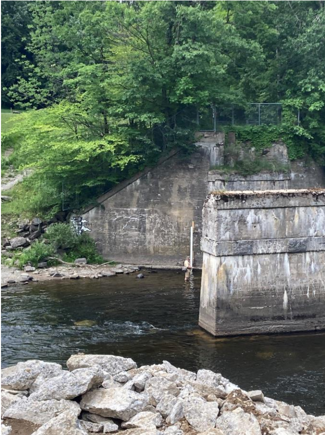
Trestle Pool site with central pier existing facing the north abutment and south abutment partially removed
