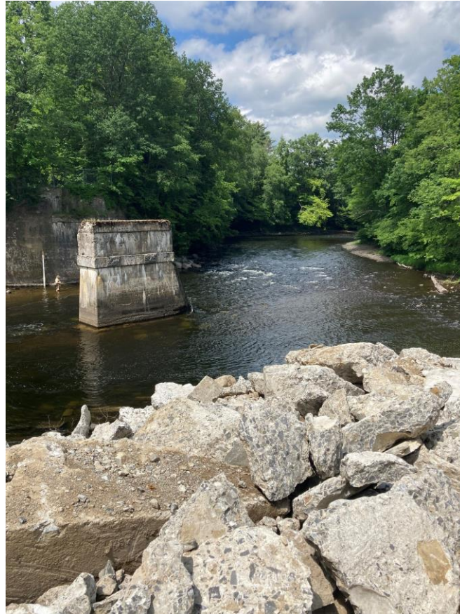
Trestle Pool site with central pier existing facing the north abutment and south abutment partially removed
