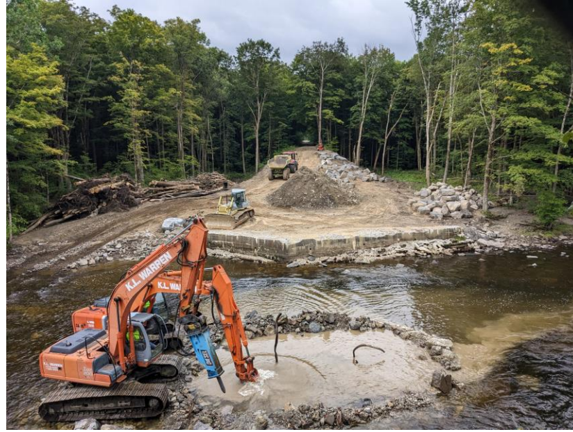
Removal of central pier facing south
