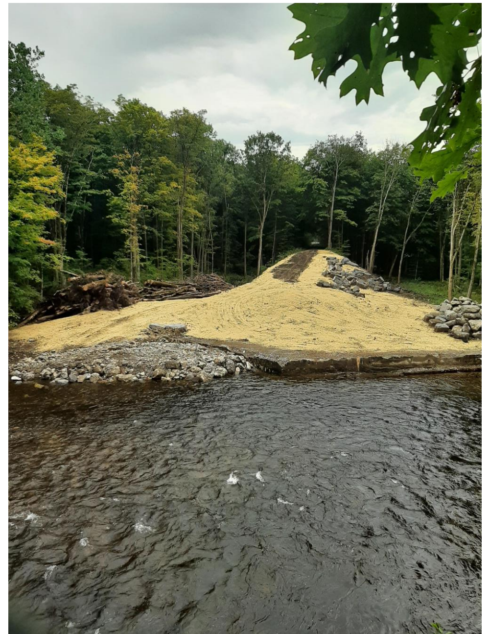
Restoration facing South
