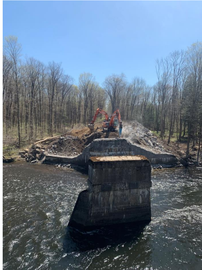
Removing the abandoned railroad grade and south abutment April 2023
