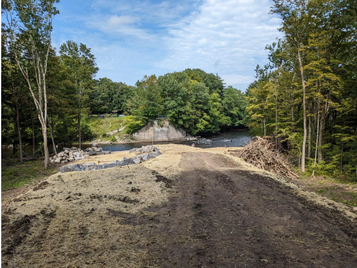
Restoration facing north abutment
