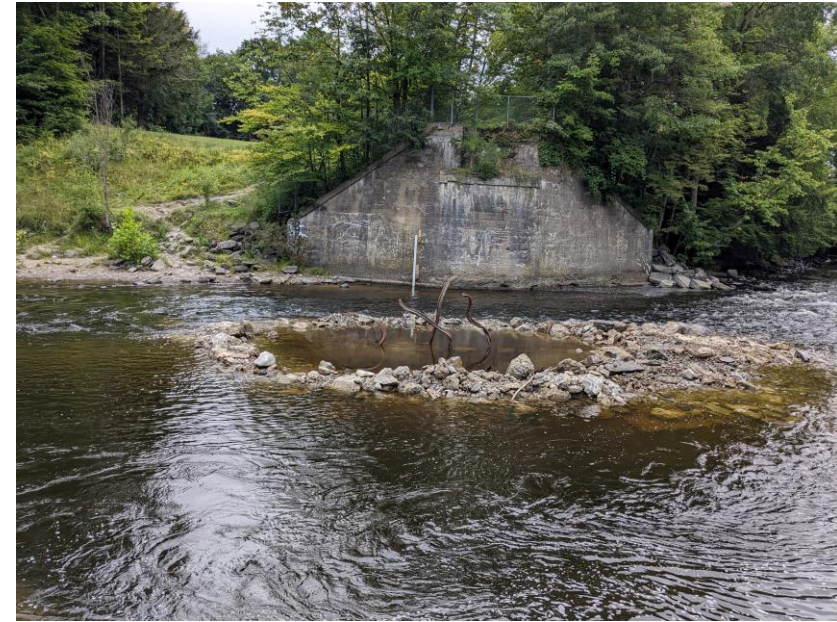
Central pier removed facing north abutment
