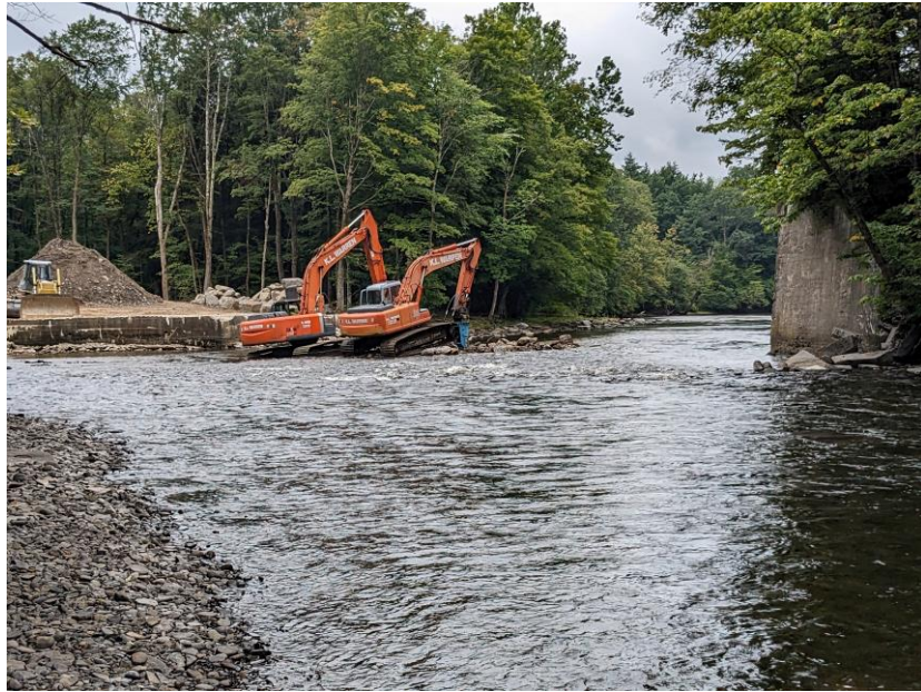
Upstream of site
