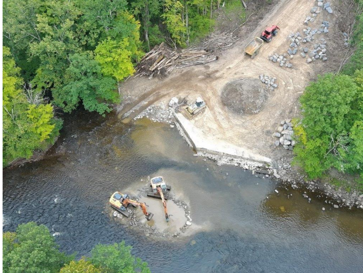
Aerial view of central pier removal and south abutment August 2023
